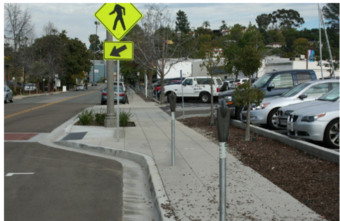
Curb extensions at mid-block crosswalks can create shorter and more visible crossing opportunities.
