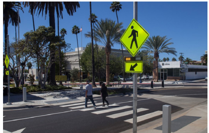
A marked crosswalk with RRFB indications creates a significantly safer environment.
