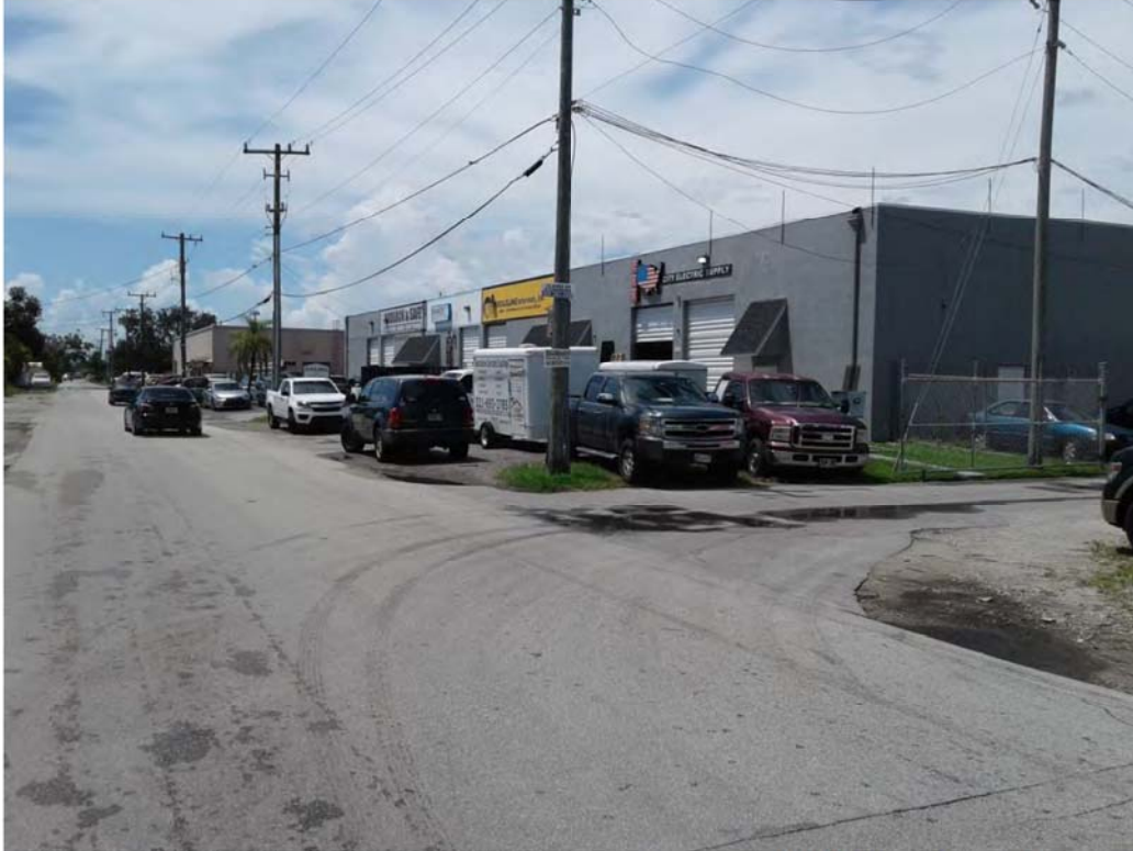
Industrial facilities along SW 70 Avenue between SW 8 Street and 9 Street
