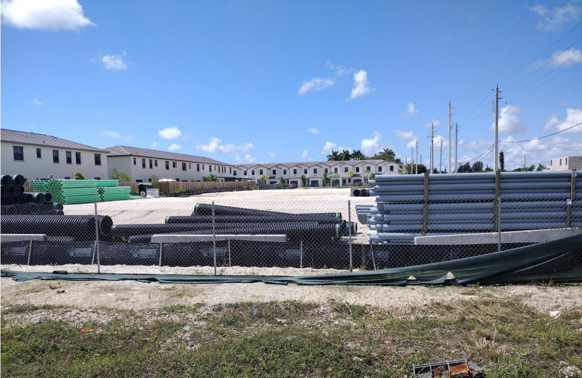
Application site looking south from the intersection of SW 132 Avenue and SW 232 Street
