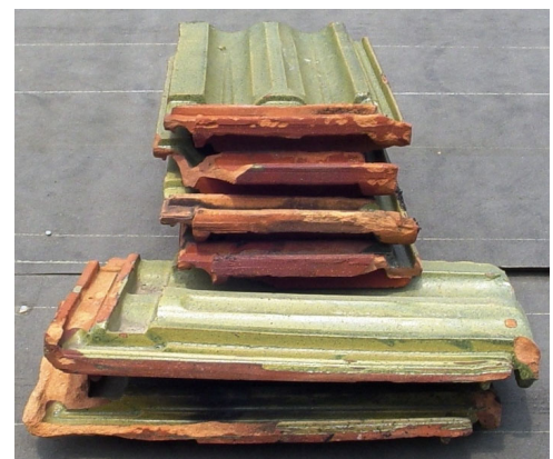
Side View - Staged Tiles (Slope ↓)
