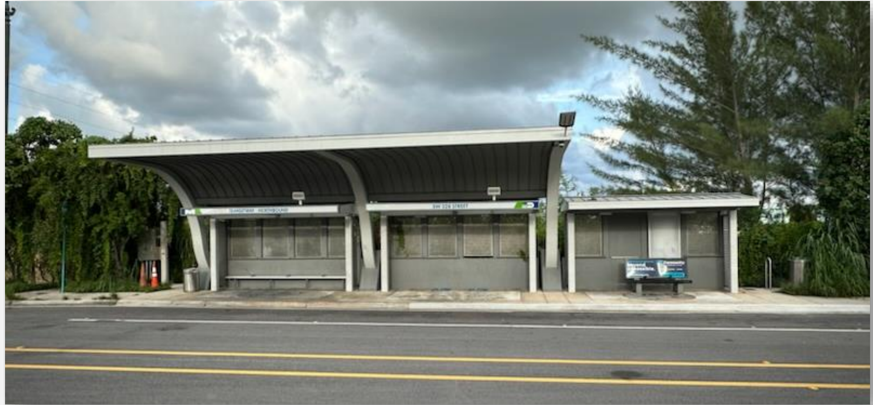
Refurbishment of exiting Bus Shelters
