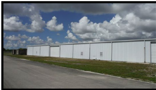
Packaging Facility Prior to Redevelopment
