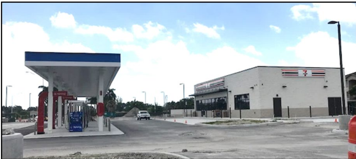
Completed Gasoline Station and Convenience Store
