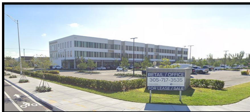
Completed Dolphin Professional Site
