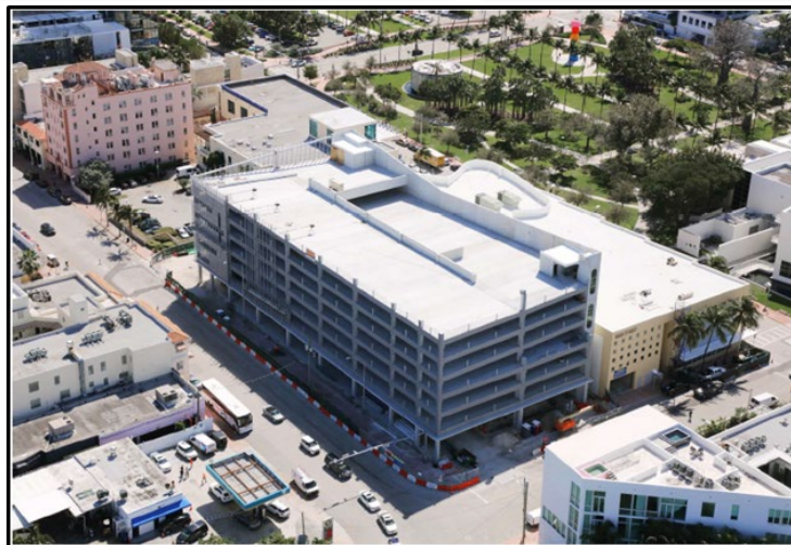
Completed Collins Park Garage
