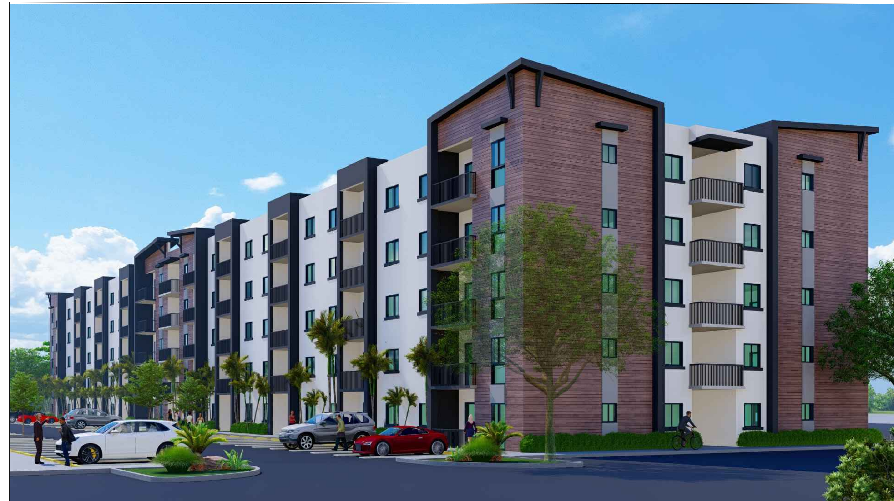
RIGHT CORNER VIEW
