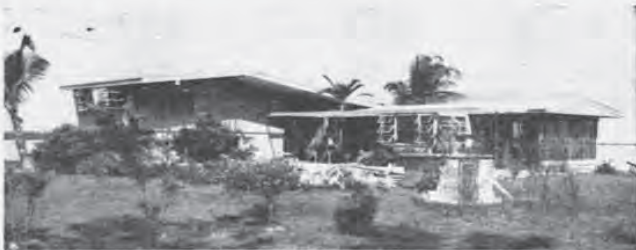
A terrace was built up from fill to allow this split-level house to get best view of the bay beside it.
