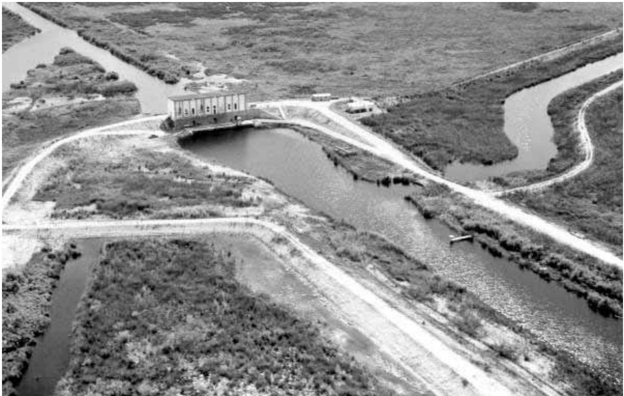
Aerial view of canal and pumping station in flood control district : Everglades, Florida , State Archives of Florida, Florida Memory, Department of Commerce Collection, c. 1960
