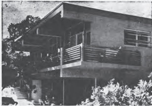
Bedroom wing, the second level of this house, is above a carport and storage area on ground level.
