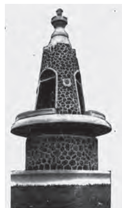
Irons Manor Fountain (1925), Miami-Dade County Historic Site, from Denis Berend, "The City Shrank in Size but Grew in Stature," Miami News , April 12, 1959
