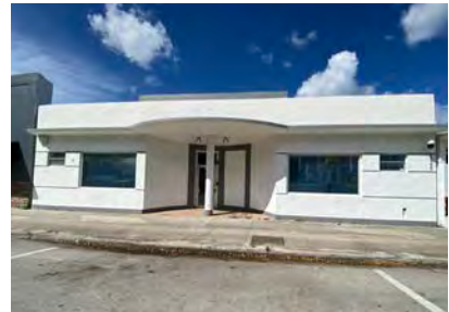
Commercial Building , 1549 NE 123rd St (1957)
