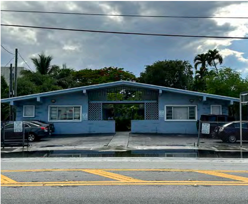
Garden Apartments , 12326 NE 6th Ave (1959)
