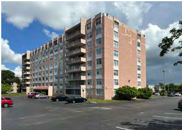
Center Court Apartments, 14695 NE 18th Ave (1971)
