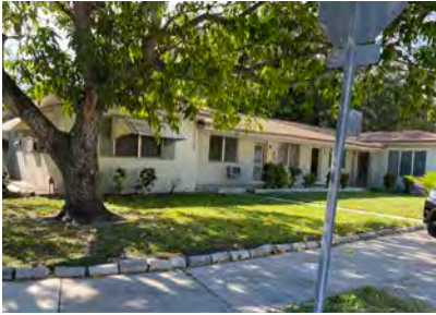
Garden Apartments , 12100 NE 7th Ave (1955)
