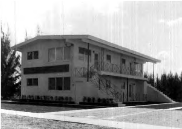
Apartment Complex (1956), Miami-Dade County, 1956
