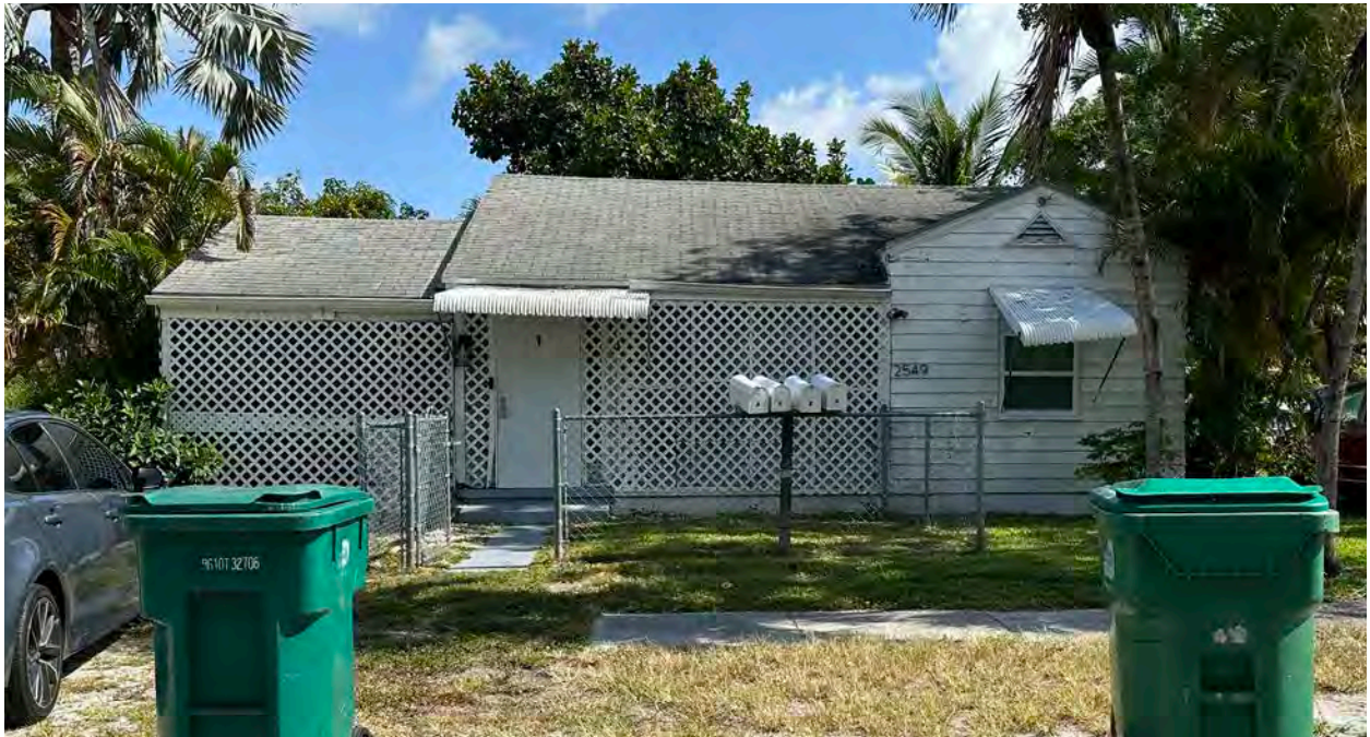
Home, Harriette Park No 2 Amd (1934)
