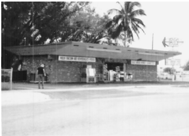
Commercial building, 13095 W. Dixie Hwy, Miami-Dade County, 1968
