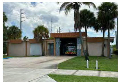
North Miami East Fire Station , 13000 NE 16th Ave (1963)
