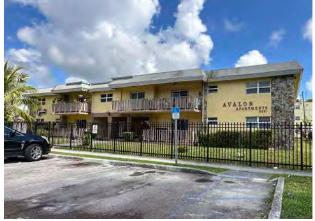
Avalon Apartments, 2251 NE 170th St (1969)
