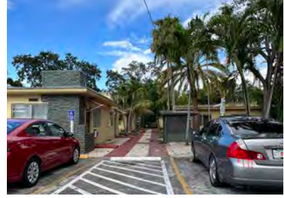
Garden Apartments , 12209 NE 6th Ave (1955)
