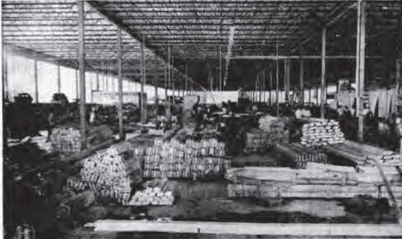
THIS WING OF ADAMS ENGINEERING CO.'S NEW OJUS PLANT IS 460 FT. LONG BY 125 FT. WIDE
