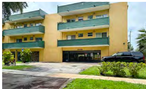
Moonraker Condominium , 1975 NE 135th St (1972)
