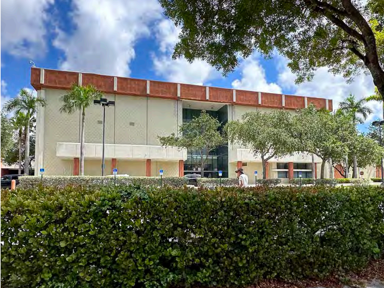
163 Street Plaza Mall, 1205 NE 163rd St (1957)
