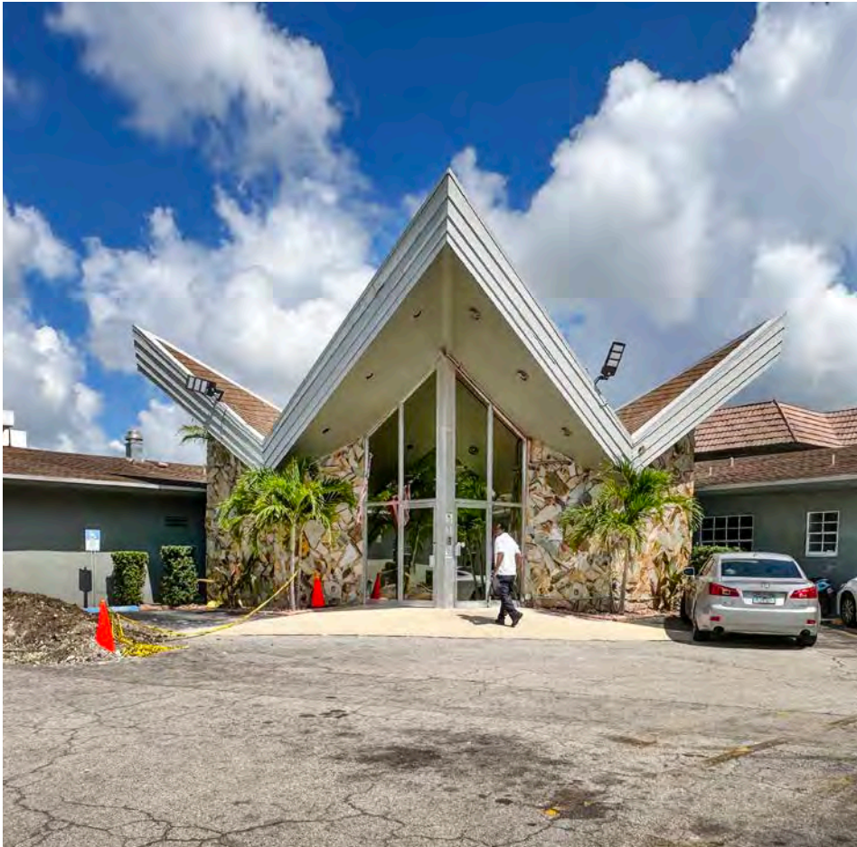
Royal Glades Nursing Home , 16650 W Dixie Hwy (1963, current Serenity Bay Nursing & Rehab)
