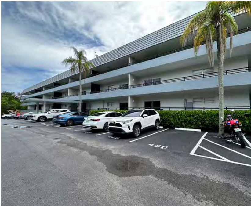
Lakeside at Biscayne Gardens, 1700 NE 133rd St (1968)
