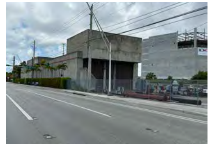
Miami Dade Water and Sewer , 15500 Biscayne Blvd. (1975)
