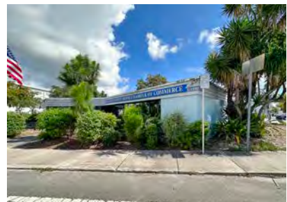
Greater North Miami Chamber of Commerce, 13100 W Dixie Hwy (1952)
