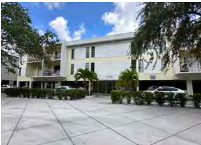
Rofalex Inc – Apartments, 1755 NE 164th St (1971)
