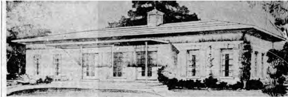
BUILT BY MEMBERS who have contributed their weekends and spare time for more than a year is this American Legion building for the J. Frank Cavanaugh Post No. 67, Arch Creek Estates, located on the Dixie highway just outside of North Miami. Designed by Architect A. L. Klingbeil, the structure, nearing completion, consists of a large assembly room, game room, auxiliary room and rest and storage rooms.
