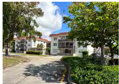
Oxford Court Condos, 13655 NE 10th Ave (1968)
