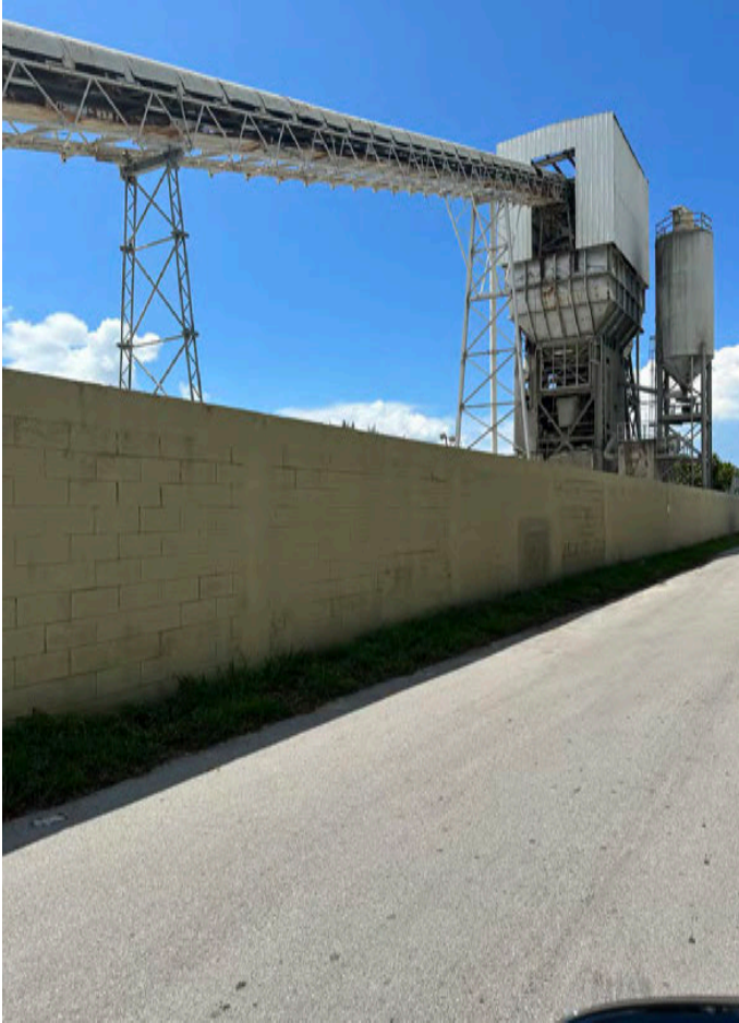
Cement plant – Cemex, 2001 NE 146th St (1974)
