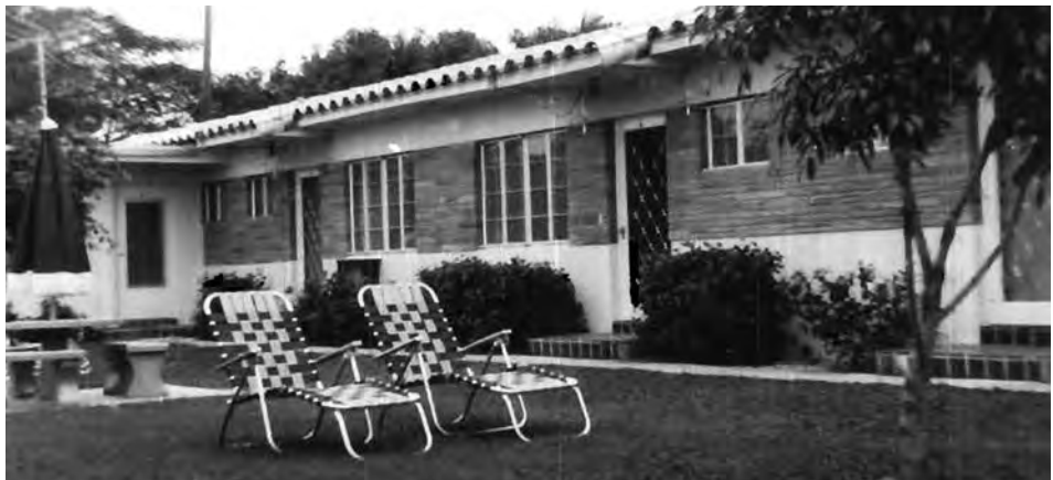
Apartment Complex (1951), Miami-Dade County, 1958
