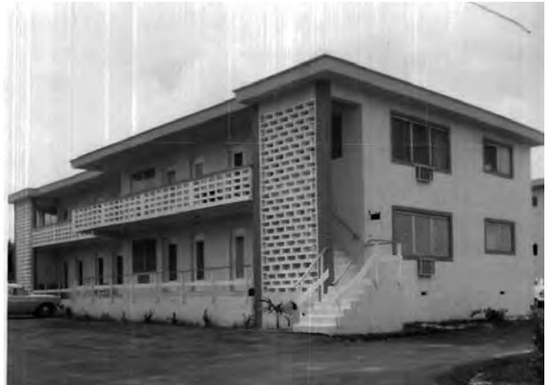
Apartment Complex (1958), Miami-Dade County, 1959
