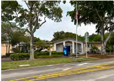
El Portal Village Hall , 500 NE 87th St (1949)
