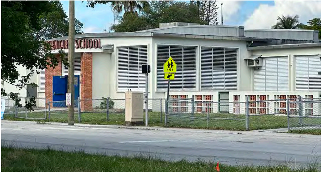
Fulford Elementary School, 16140 NE 18th Ave (1925)
