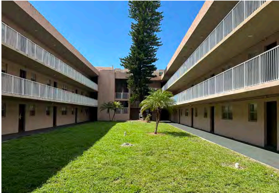
Center Court Apartments , 14695 NE 18th Ave (1971)
