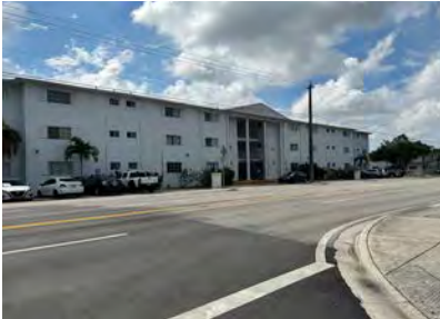
The Whitehouse Condo , 13700 NE 6th Ave (1964)
