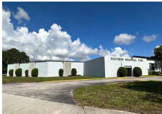
Southern Memorial Park, 15000 W Dixie Hwy (1941 - 1975)
