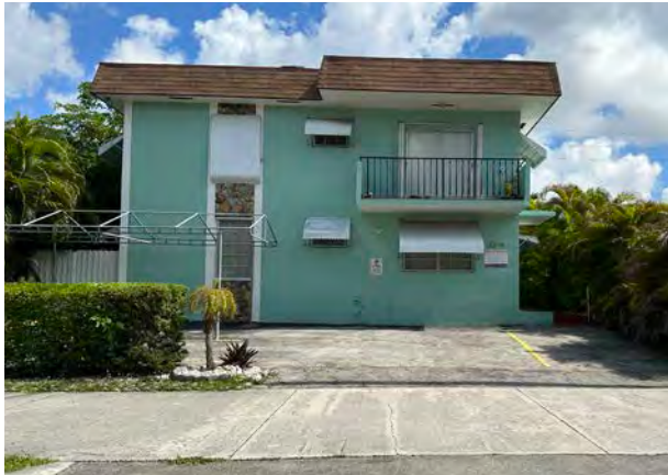
Apartments, 2379 NE 172nd St (1969)
