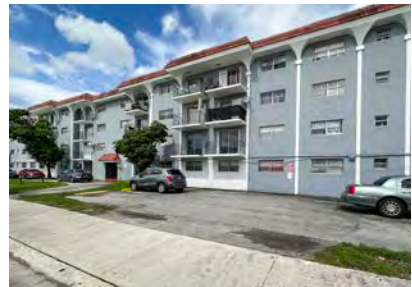
Tropical Terrace Condo, 13725 NE 6th Ave (1971)
