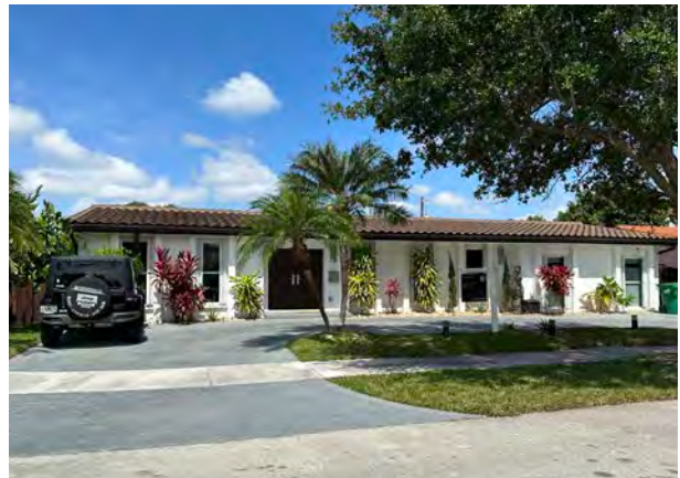
Home, Skyknoll Ests Replat (1971)
