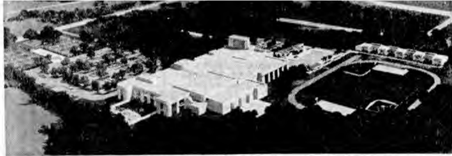
Phase One Half-Way Completed at Community Center ... total project cost set at $5.5 million
