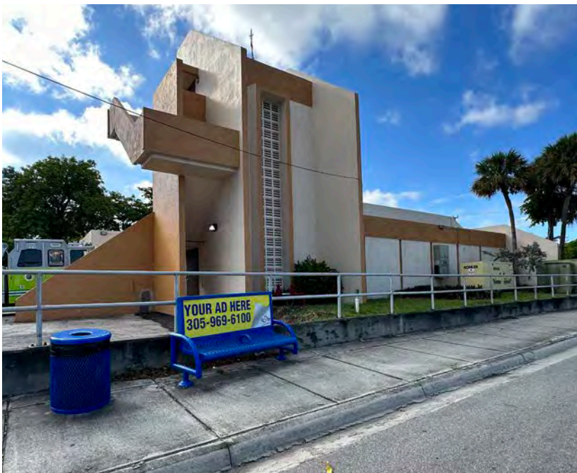
Miami Dade County Fire Rescue Station 22 , 15655 Biscayne Blvd (1976)
