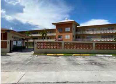
Sutton House Apartments , 11855 NE 19th Dr (1963)
