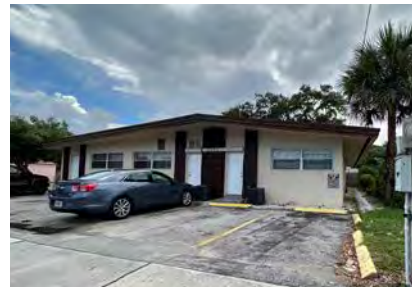
Garden Apartments , 13200 NE 6th Ave (1960)
