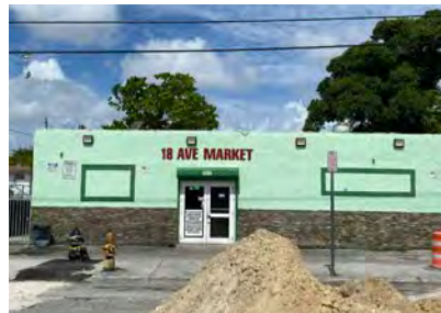
18 Ave Market , 6606 NW 18th Ave (1969)
