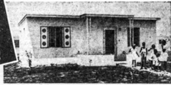
Typical modern home... designed for all-electric living.
