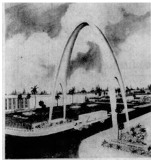
ARCH OF INDUSTRY is scheduled to be put in place this week William Webb's Sunshine State Industrial Park on the Palmetto Bypass. The 120-foot arch has been constructed by Gemco International, Inc., of Fort Lauderdale and is made of reinforced concrete. A plastic material with marble chips is sprayed on the surface to give it a golden, glittering surface. The spray process was developed by Richard A. Weir and Scott Campbell, both of Fort Lauderdale.
