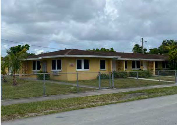
Solivette Low Rent Housing Project, 6321 NW 25th Ave (1962)
