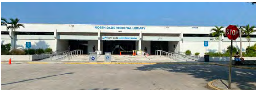
North Dade Regional Library, 2455 NW 183rd St (1979)
