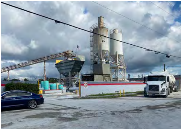
Supermix - Perrine Plant, 9795 SW 170th St (1959)
