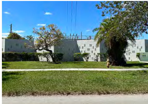
FPL Electrical, 12250 SW 82nd Ave (1968)
