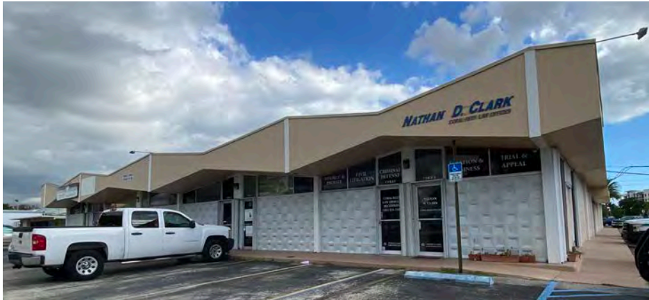
Commercial building, 17641 S Dixie Hwy (1960, Current Nathan D. Clark, Esq. - Coral Reef Law Offices, PA)
