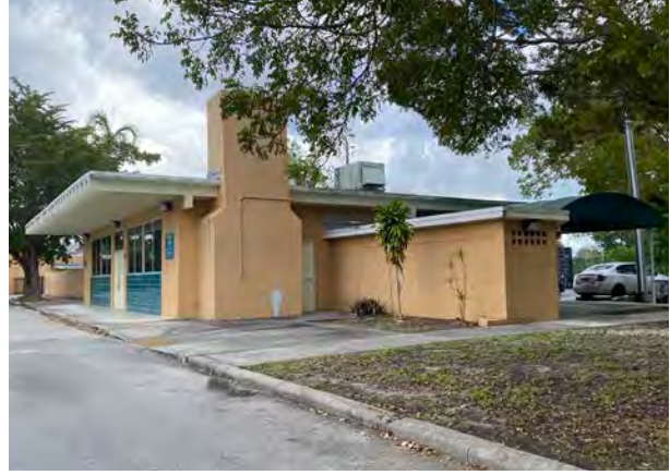
West Perrine Senior Center, 17801 Homestead Ave (1961)
