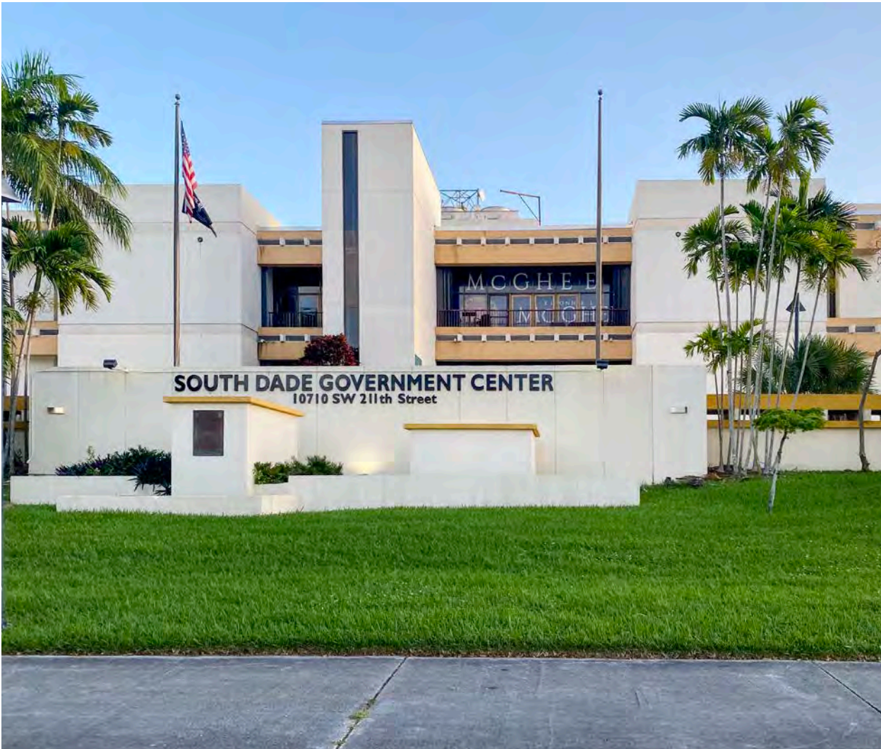
South Dade Government Center, 10710 SW 211th St (1970)
