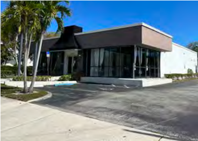
Commercial building, 8935 S Dixie Hwy, Miami, FL 33156 (1981, current Casa Contemporanea)
