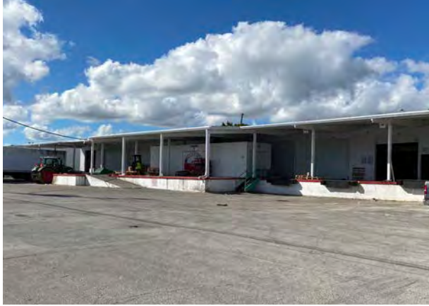
Florida City Industrial Site, 300 N Krome Ave (1940)
