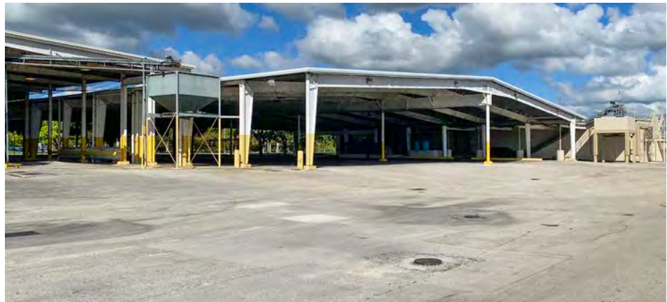
Florida City Industrial Site, 300 N Krome Ave (1940)
