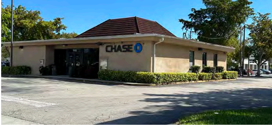
Bank , 15101 S Dixie Hwy (1967, current Chase)
