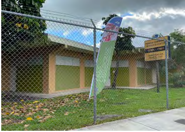
West Perrine Senior Center, 17801 Homestead Ave (1961)
