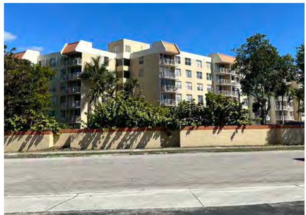
Village at the Falls Condos, 13100 SW 92nd Ave (1974)
