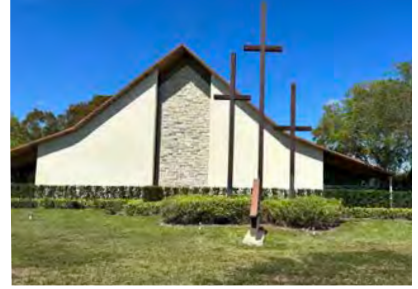
Kendall Presbyterian Church, 8485 SW 112th St (1958)
