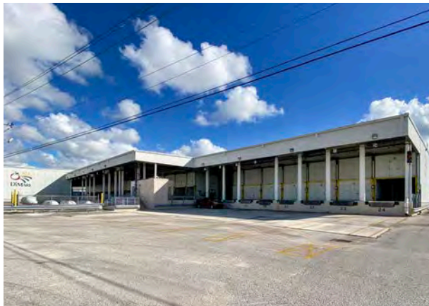
Di Mare 48 SW 1st St, Industrial Addn No (1988)
