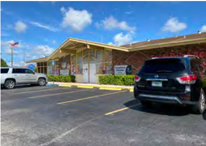
Commercial building, 27835 S Dixie Hwy (1979, current South Point Academy)
