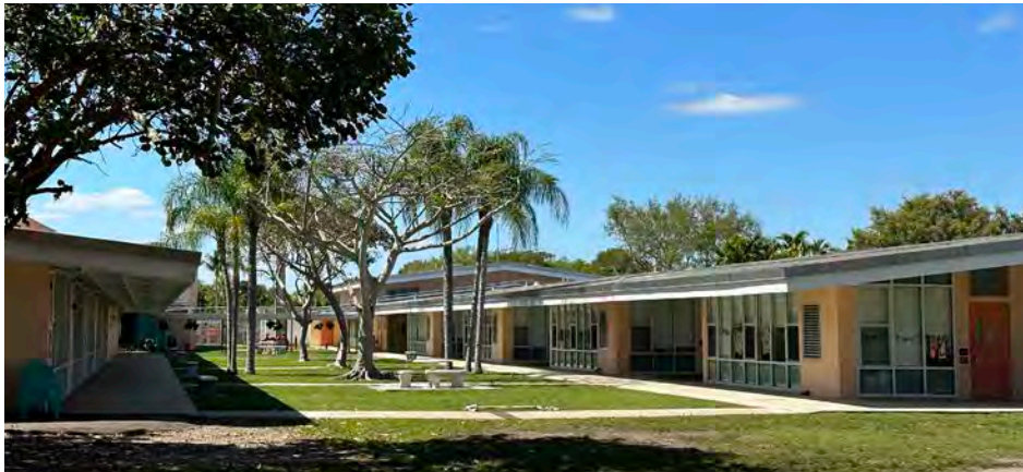
Vineland k-8 center Elementary School, 8455 SW 119th St (1959)
