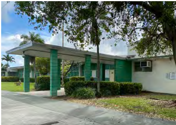
Leisure City K-8 Center, 14950 SW 288th St (1960)
