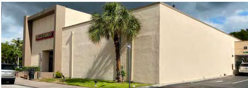
Coral Gables Federal Savings and Loan Association, 17401 SW 97th Ave (1958, Current Wells Fargo)
