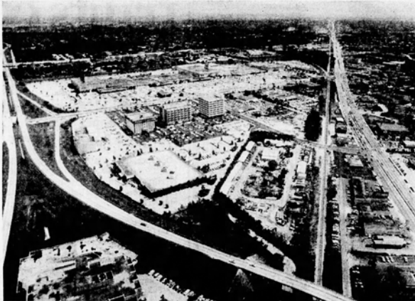
Dadeland is located at the junction of U.S. 1 and the Palmetto Expressway ... skeptics said the giant mall would never pay for itself
