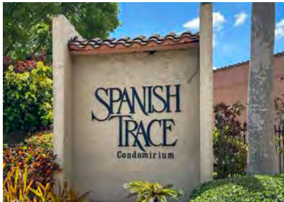
Spanish Trace Condominium, 10766 SW 88th St (1968)
