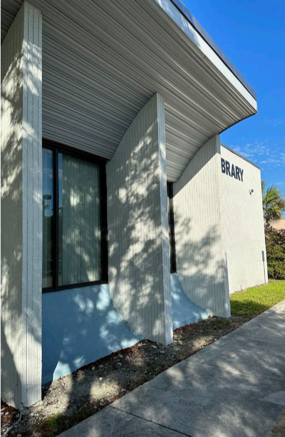
Kendall Branch Library, 9101 SW 97th Ave (1978)
