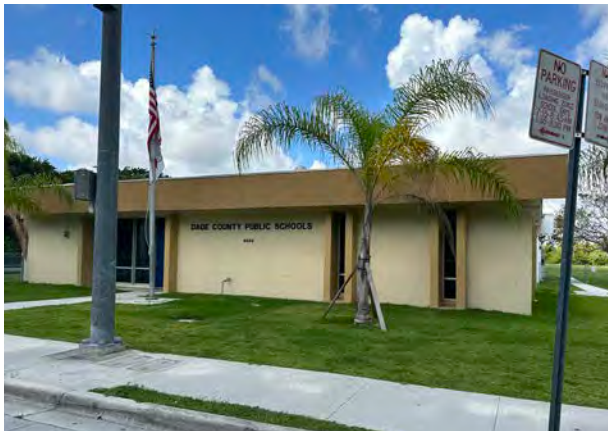
Dade County Public Schools Building, 9300 SW 79th Ave (1956)
