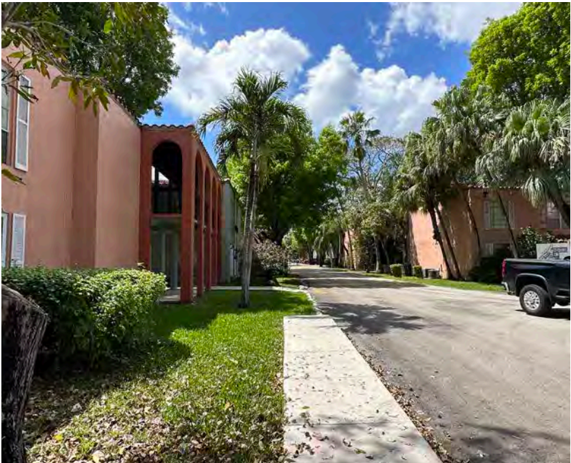
Spanish Trace Condominium, 10766 SW 88th St (1968)
