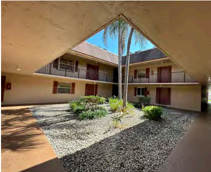
Pine Grove Condominium, 11251 SW 88th St (1969)
