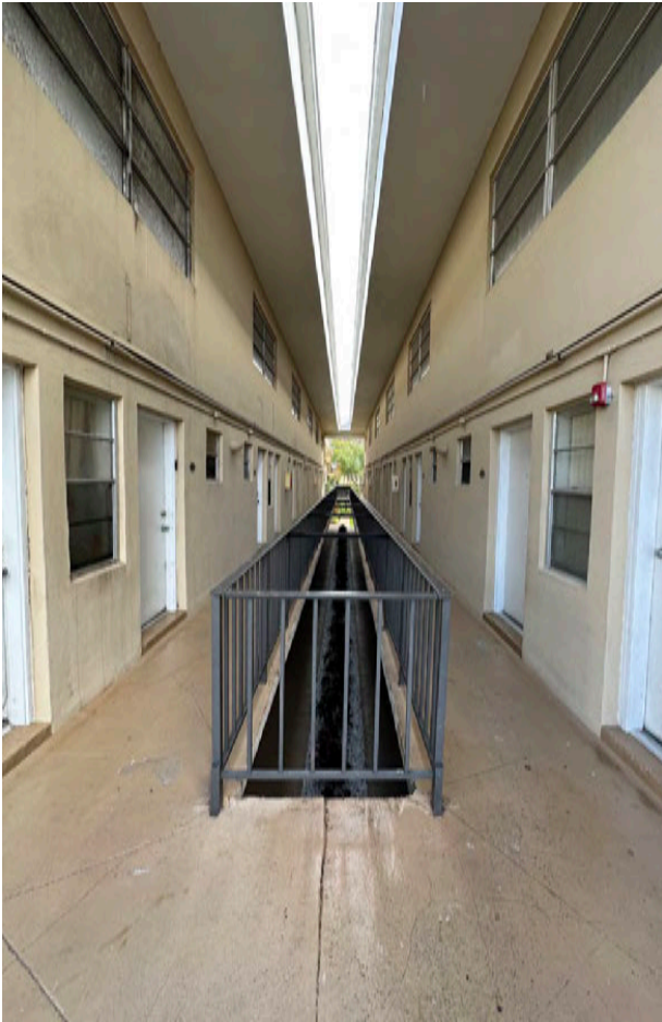
Colony at Dadeland Apartments, 9345 SW 77th Ave (1967)
