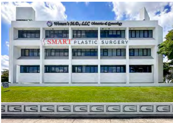
Capital Plaza , 10700 SW 88th St (1982, Current Office Building)
