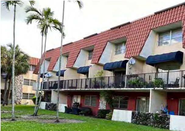
Colony at Dadeland Apartments, 9345 SW 77th Ave (1967)
