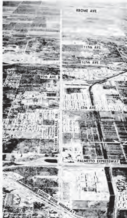
N. KENDALL DRIVE, once just a two-lane road through a vast undeveloped South Dade area, is now one of the fastest growing areas in
