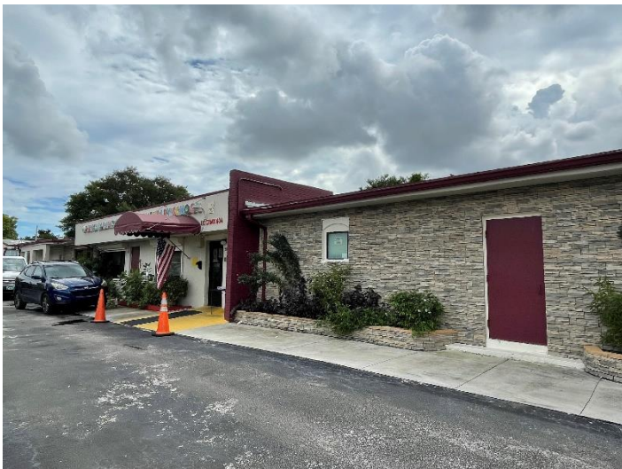
Former Jackson's Toddle Inn Building, today Sheyes Learning Center and Elementary School, October 2022.
