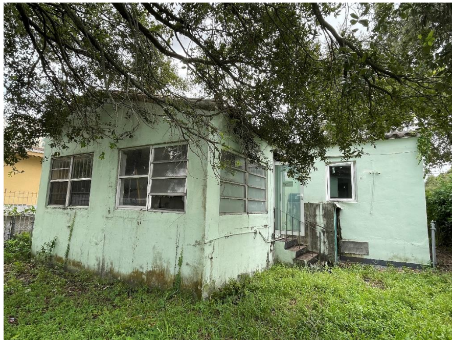
Rear/north elevation, October 2022.
