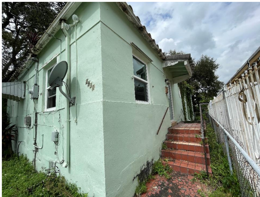
Southeast corner, façade and side/east elevation with main entry, October 2022.
