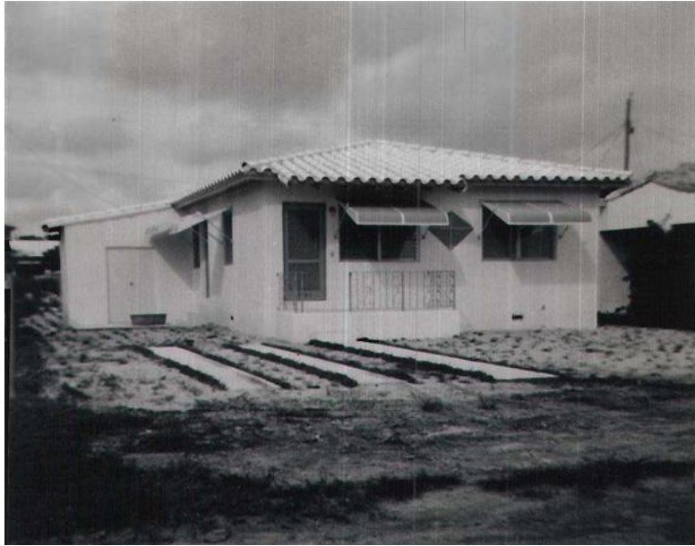
Former Jackson-Mosley Home, 3021 NW 48 Terrace, c.1960. 18
