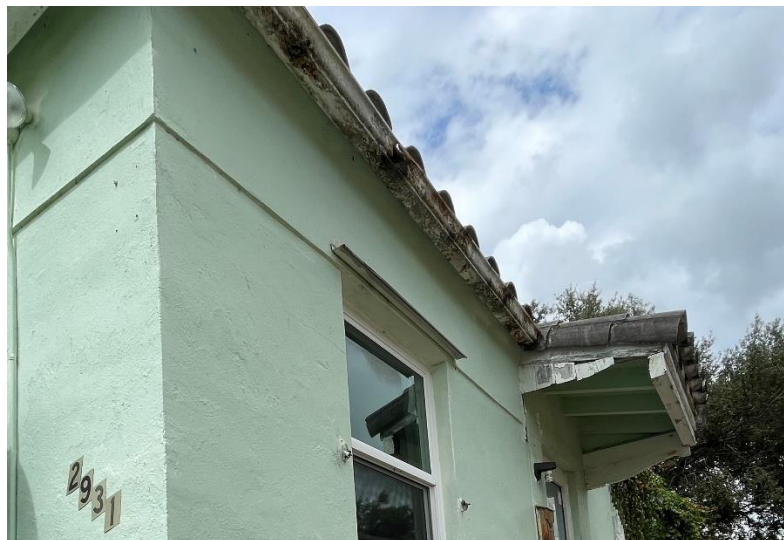
Concrete barrel tile roof and entry overhang.
