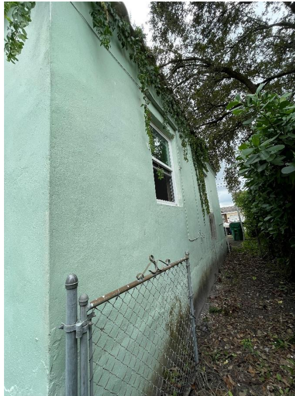
Side/west elevation, October 2022.
