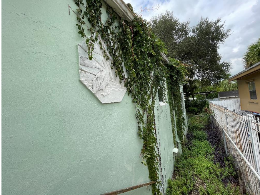
Side/east elevation just beyond main entry, October 2022.
