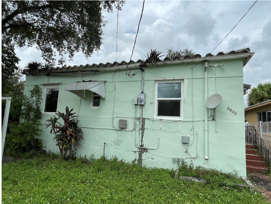
Facade/south elevation, October 2022.
