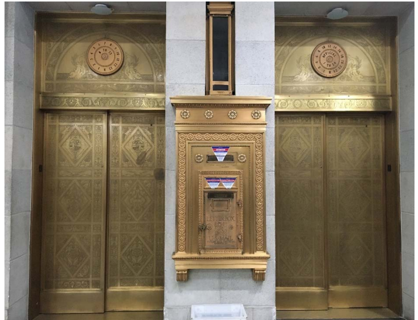
View of two of the original etched bronze elevator doors in the lobby with the original bronze mailbox and tube above, January 2020. (Photo courtesy Office of Historic Preservation.)
