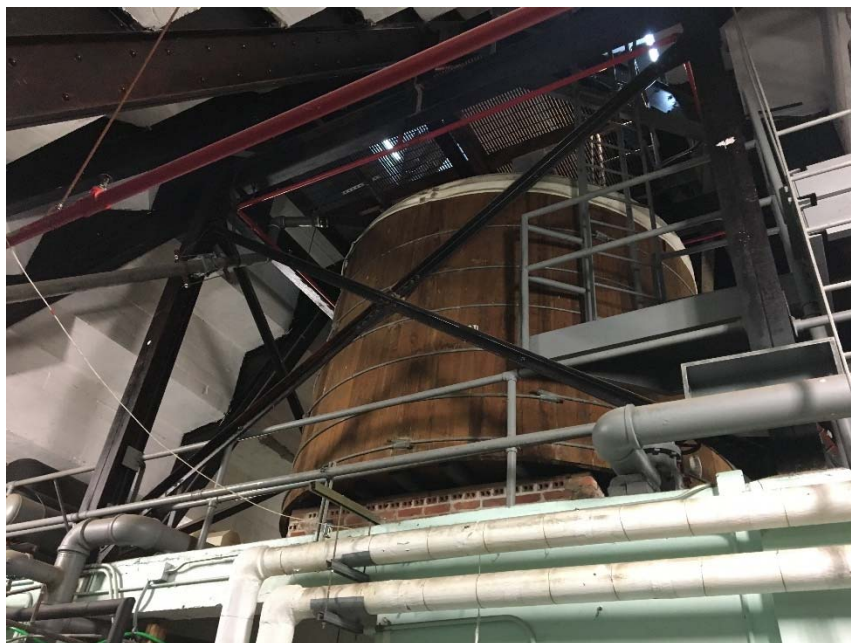
View of the wooden water tank housed in the ziggurat roof, September 2018. (Photo courtesy Office of Historic Preservation.)
