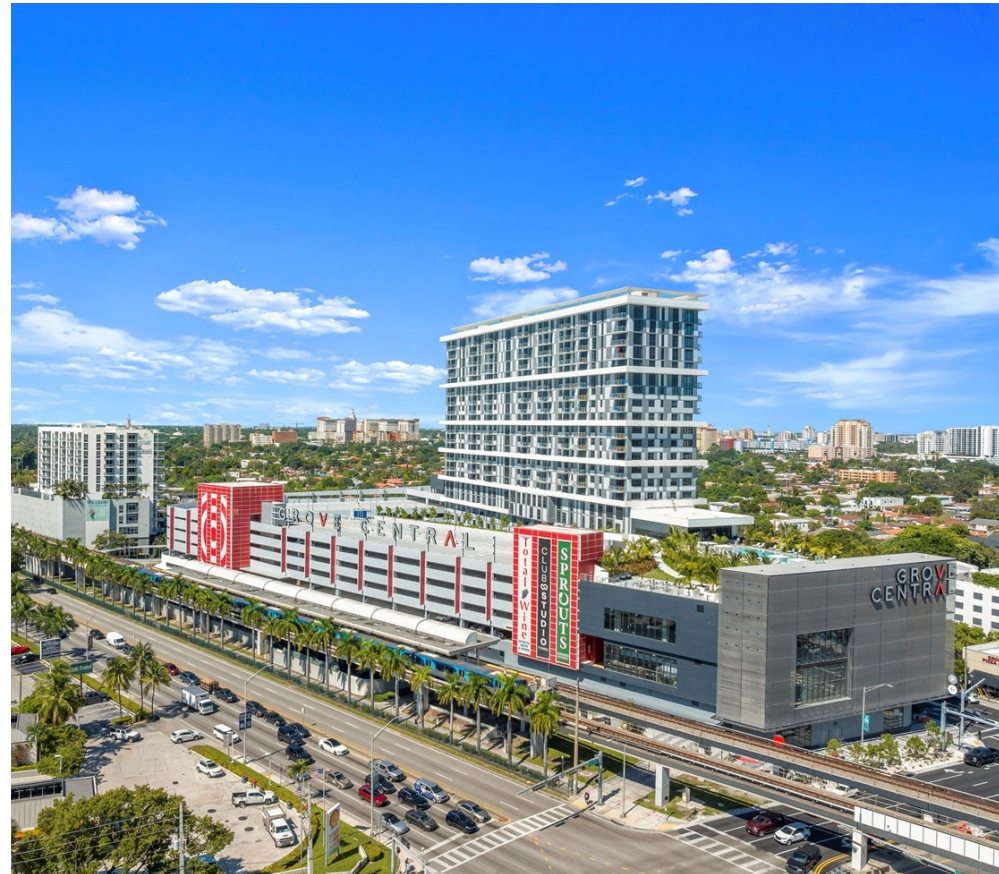
Grove Station Coral Gables Station Douglas Road Station
