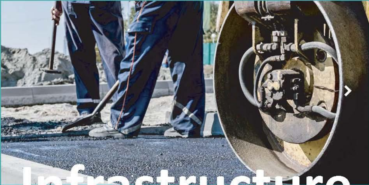
Image: Redevelopment Support/ Economic Incentives: Tax Increment Recapture, Infrastructure Grant & Community Benefits Agreements, North Miami, Florida. (Source: North Miami CRA)
