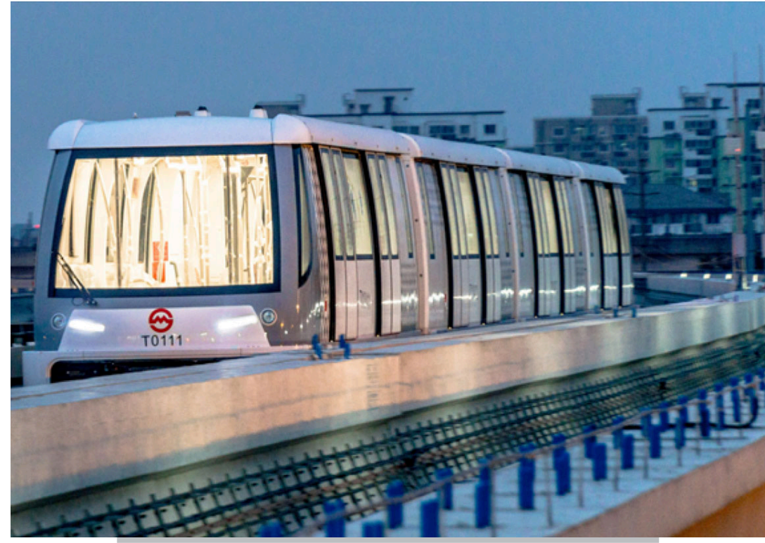
Automated People Mover (APM)
